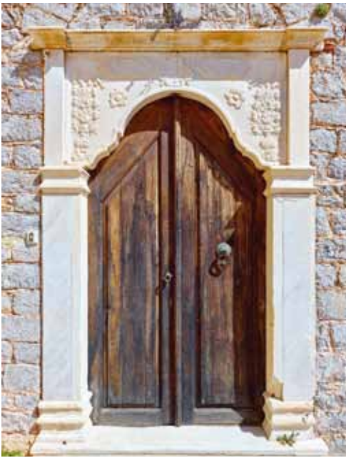
Entry to upper terrace
