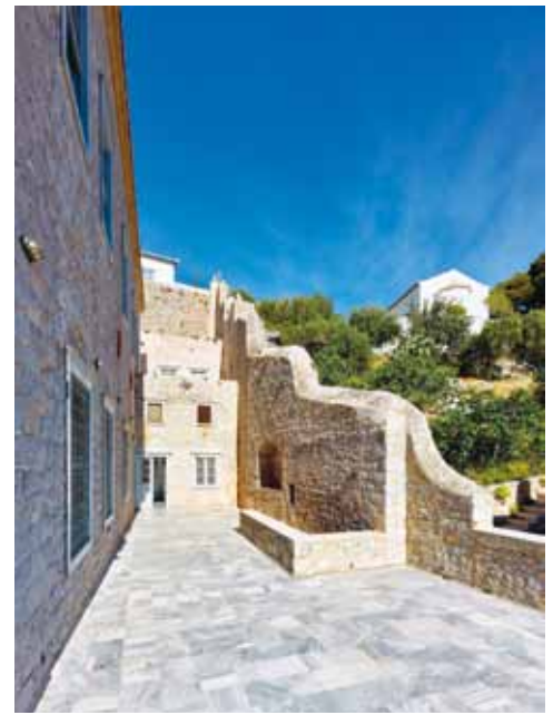
Terrace on the second floor
